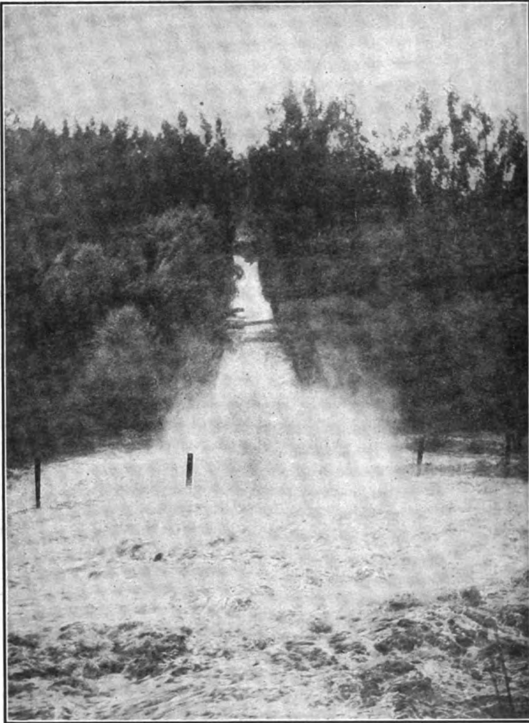
HOW THE WATER OVERFLOWS AT TIMES FROM WASTE TUNNEL NO. 3. SAN LEANDRO RESERVOIR
